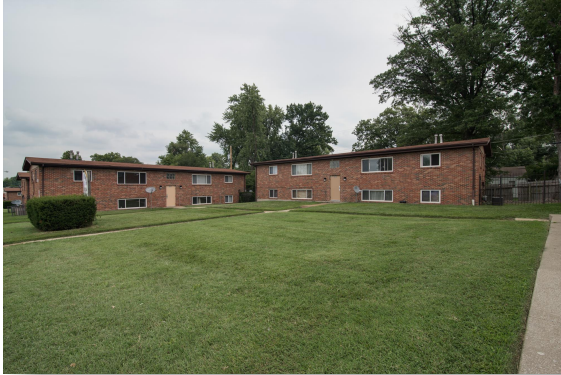
Solid Brick Buildings with green space
