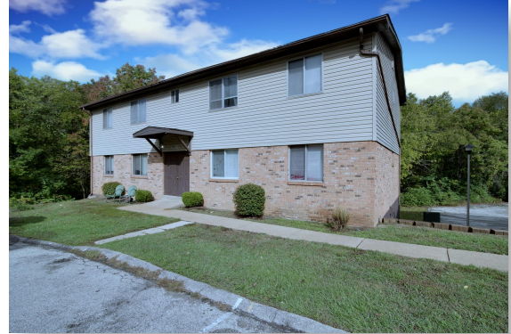
Well Maintained Buildings
